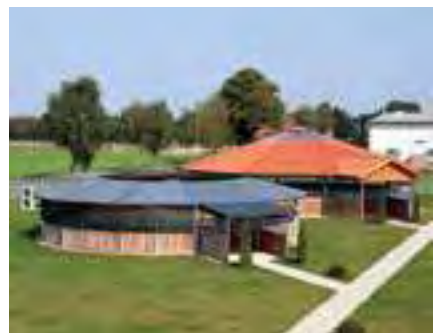
2014 Completion of the Röwer & Rüb show park with over 7000 m 2 of exhibition space.
