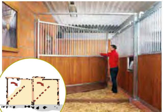
Hinged partitions permit manure removal from entire rows of stalls.
