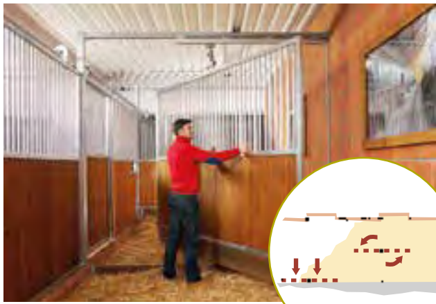
1 The hinged and sliding partition is suitable for stalls that are deeper than wide.
