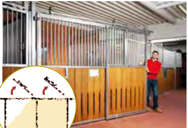
If individual stalls are cleaned from the front with an articulated arm, the hinged front wall is an ideal solution.
